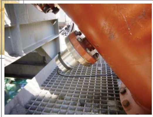
Large pipe installation v
