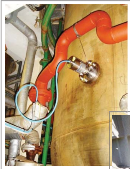
< Batch resin reactor installation
