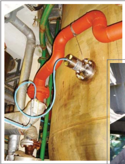
< Batch resin reactor installation
