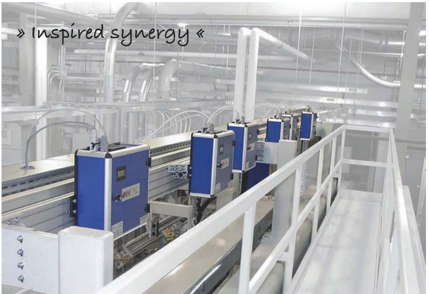
Cooperation Brückner ServTech & OCS
